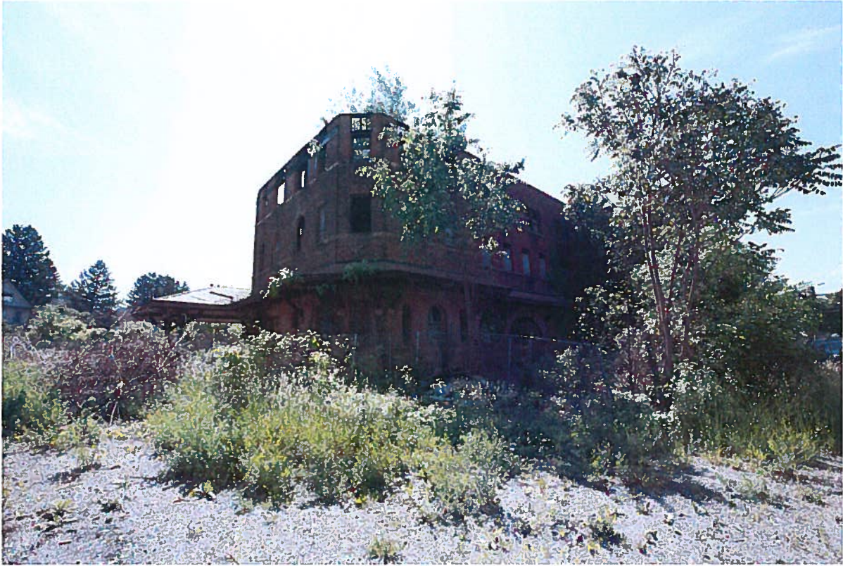
North tower view
